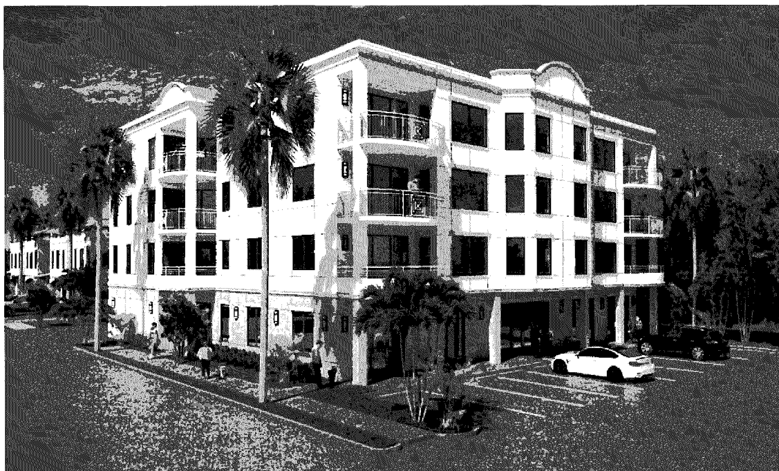
Exterior View from Southeast, looking Northwest
